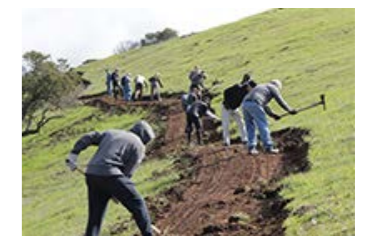
A view of trail building
